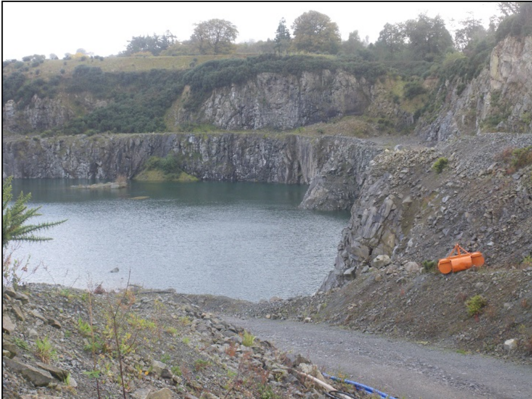
View southwards of western side of quarry, showing vertical faces and flooded quarry floor. Upper faces to right are readily accessible.
